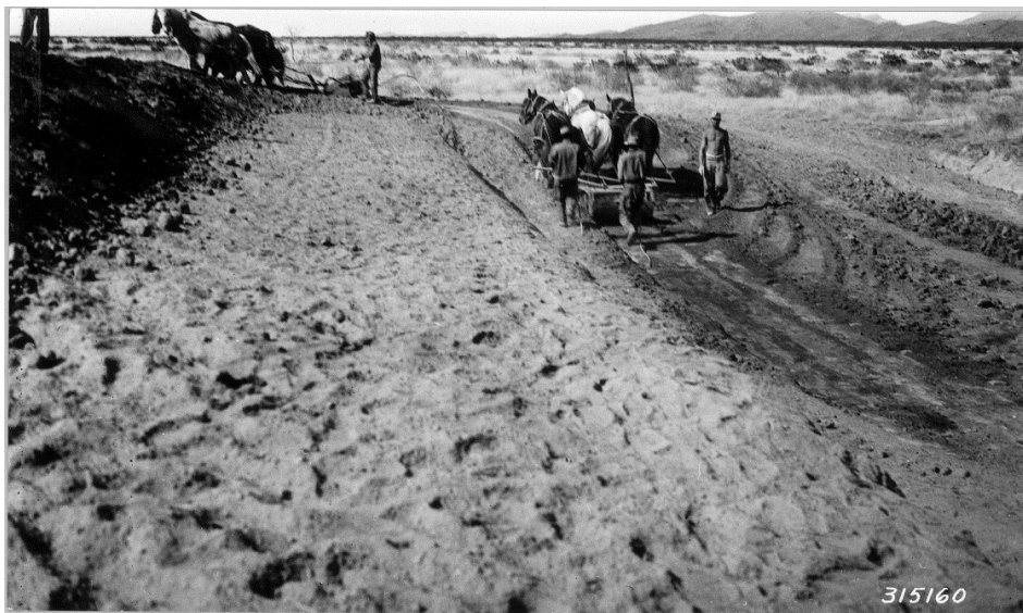
Fig. 4. Construction of stock water storage tanks at the Jornada Experimental Range using three-horse Fresno teams on Big Meadows tank by the Civilian Conservation Corps (CCC) in April 1934.
