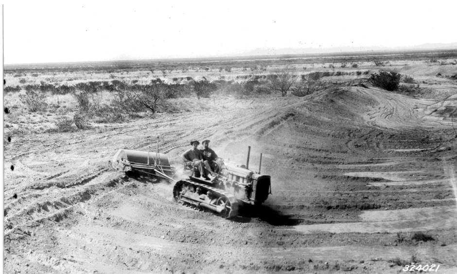
Fig. 5. Use of mechanized earth moving equipment during construction of Big Meadows tank at the Jornada Experimental Range in 1934. New equipment and the availability of the CCC labor force were some of the reasons for the revitalization of water harvesting on rangelands.
